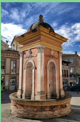
The fountain in Samatan
